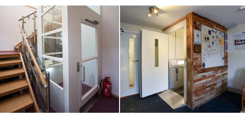
The Niche Altair internal platform lifts provide safe, efficient and smooth vertical travel up to 9 metres (6 floors). With their free-standing and self-supporting structure (requires anchoring to the building), and options for no pit and no motor room, the Altair platform lifts are both quick and easy to install.
