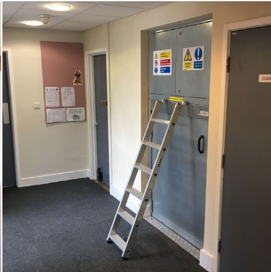
Ladder option to allow for access to the lift machinery
