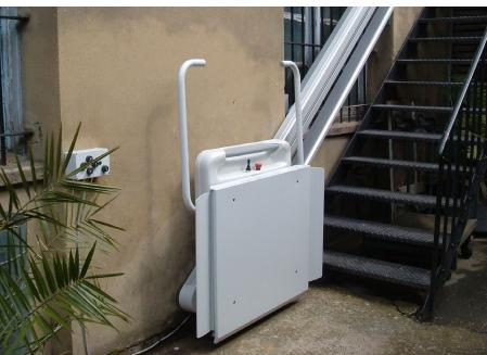
Niche Dorado Inclined Platform Lifts are designed for straight stairways, and their compact folded platforms provide a smooth ride for wheelchair users. Their fully automatic operation makes them safe and easy for passengers to utilise, with no special training or requirements necessary to operate them.
